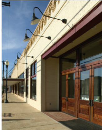
Pontotoc Chancery Annex Pontotoc, MS
